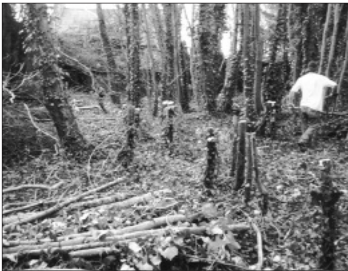
Tree felling in progress, February 2005
