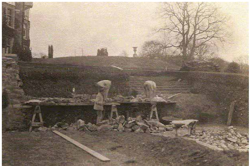
Construction of the Bodnant terraces, Images courtesy of the NT
